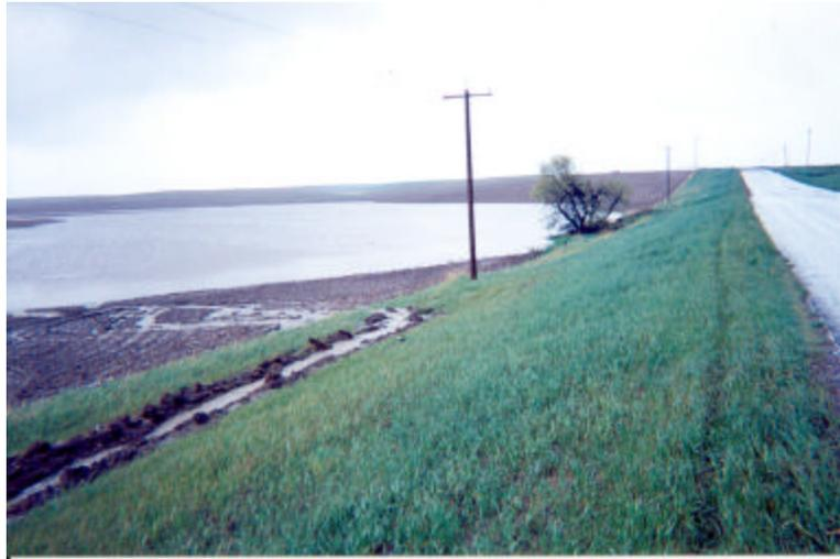
Figure 2 (a). Elevated roads: A large pool of runoff accumulates on the upslope side of an elevated road after a rare prolonged precipitation event in June, 2002. The downslope side of the road (not shown) showed no signs of runoff accumulation.
