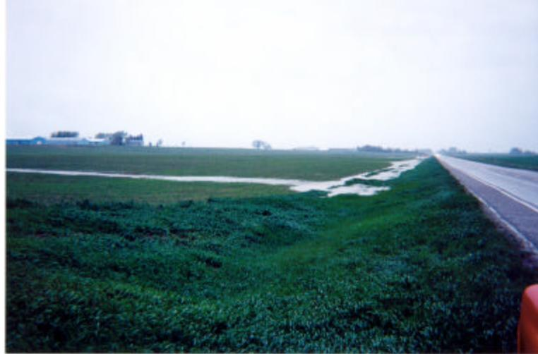
Figure 3 (a). Roadside ditches: Runoff changes its flow direction abruptly due to the presence of a road with ditches. The runoff in the picture is flowing from the field towards the road, at which point, the road imposes a ninety-degree change in direction. Thus, the roadside ditch enforces the progression of the runoff along the road perpendicular to the natural drainage pattern.
