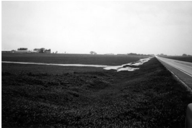
Figure 3. Runoff flowing along the topographic slope, from the field towards the road, is deflected 90° by a secondary highway. Most roads in southern Alberta are raised to reduce the potential for snowdrift during winter (Duke et al. , 2003)
