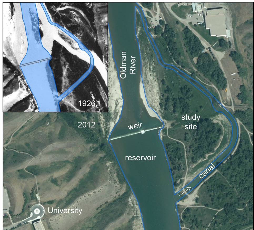
Fig. 2 Aerial photograph of the study site along the Oldman River in 2012 with an inset image from 1926
